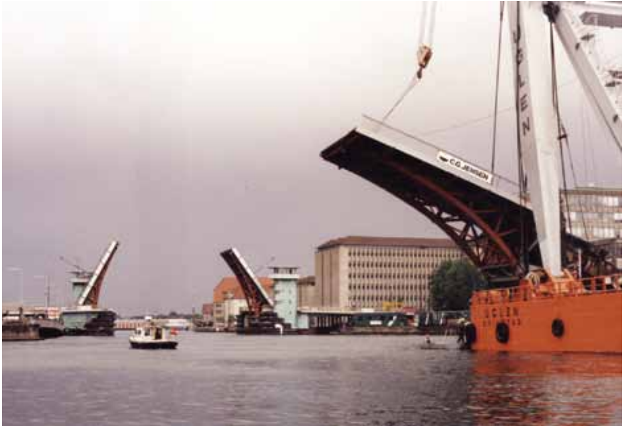
The floating crane transporting one quarter of the bascule bridge.
